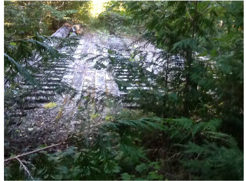
Left approach facing structure
