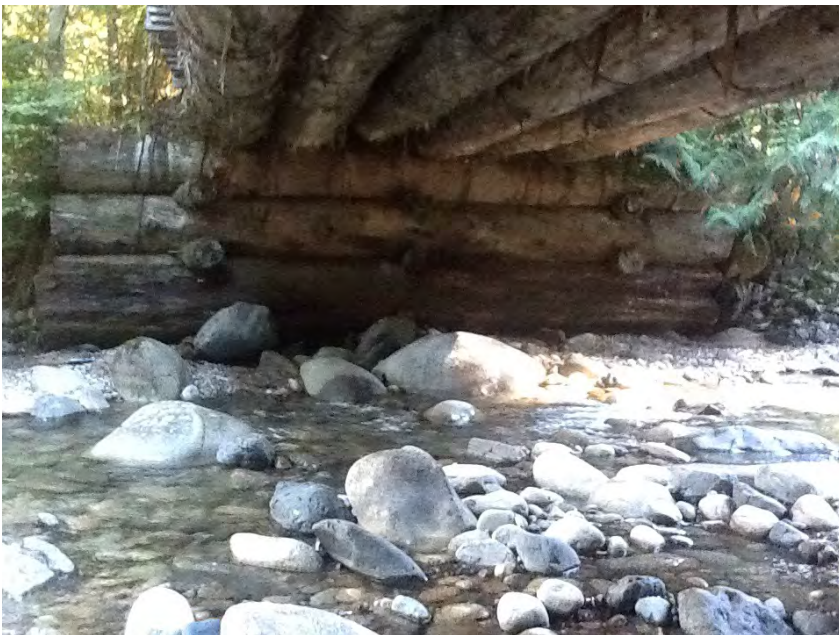
Right Bank Abutment when facing downstream
