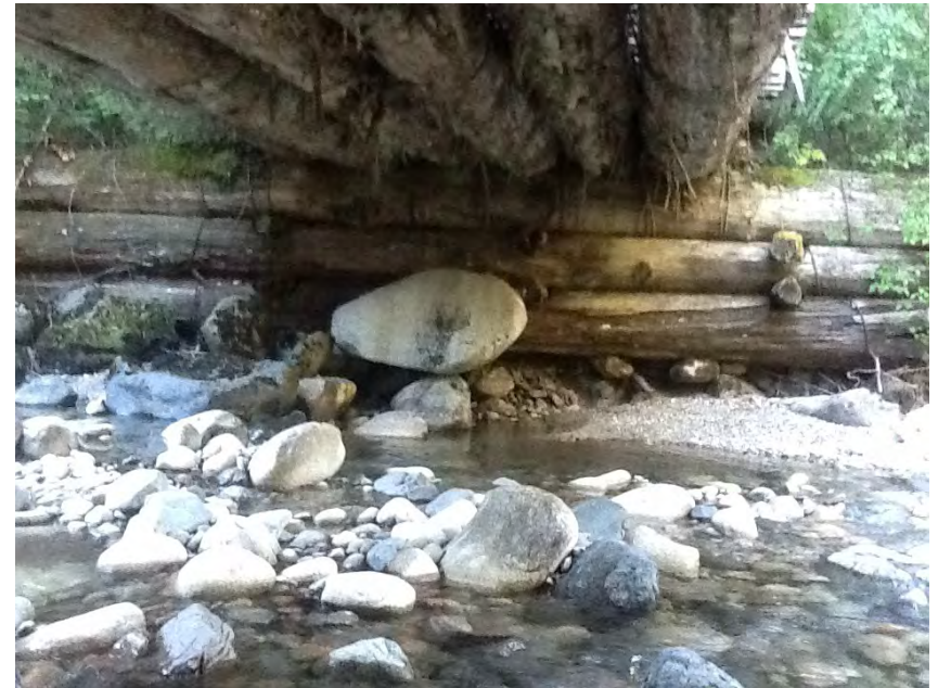
Left Bank Abutment when facing downstream
