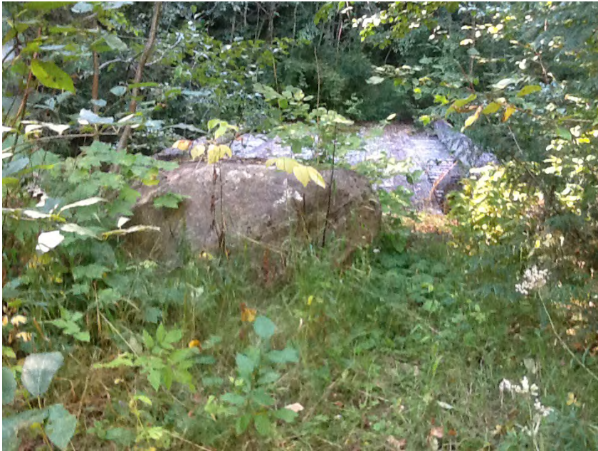
Right approach facing structure
